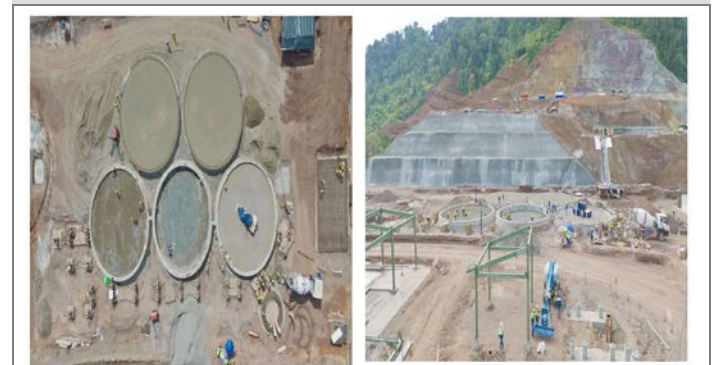
Figure 2: Processing Plant Construction
